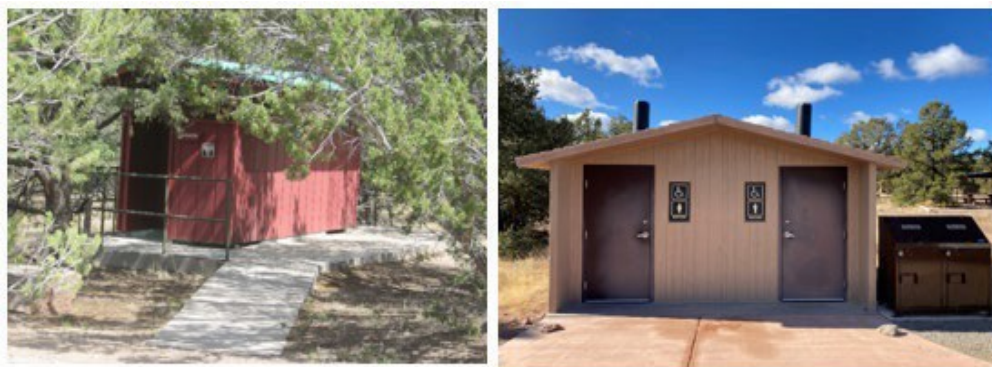
Figure 11: 2022 Vault Toilet Replacement
