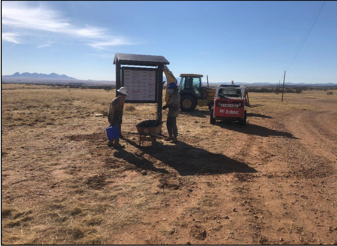
Figure 3. Installation of the Maternity Well Group Site information kiosk by BLM staff and ACE youth crews.
